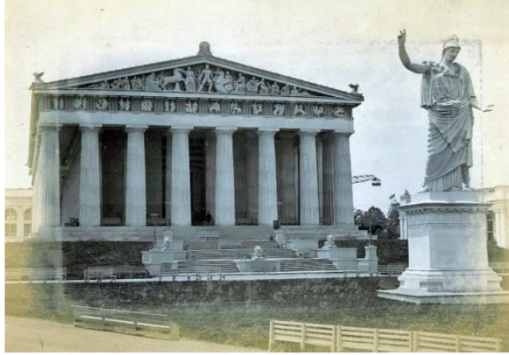
Commerce Building, Parthenon, See-Saw, and Pallas Athena
