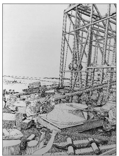
An architect inspects the piece for cracks while masons examine the dimensions, work that demands expert knowledge of geometry.
